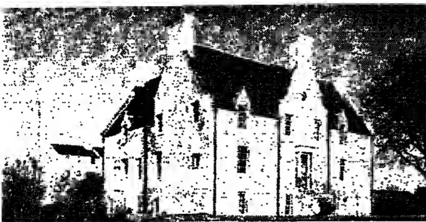
Pirig House, Bonnington Road, Edinburgh. A late example of a traditional Scottish laird's house built in 1838 in an L-shaped plan around a turpika stair for an
